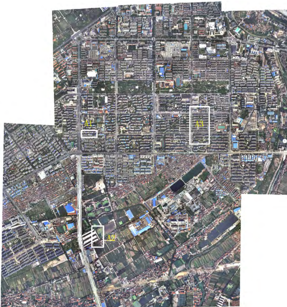
Fig. 13. Final mosaic of six images using the building map. Details of three sub areas (A1, A2, and A3) are shown in Figs. 14–16.
